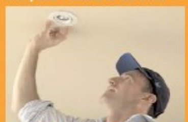
Downlight reconnected and fitted as normal with transformer outside the cover
