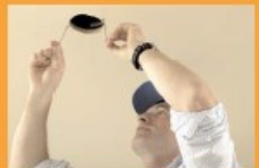
L section of wire frame clears the underside of the ceiling and fits into place – excess is removed
