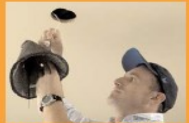
Wiring loom threaded through cover
