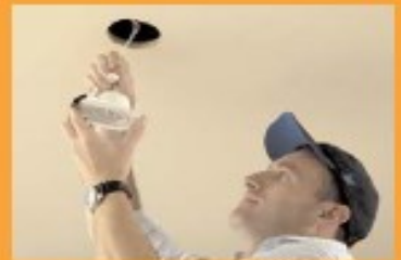
Downlight removed and supply disconnected
