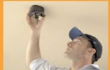
Cover fed through downlight cut-out
