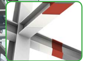
Intumescent Paint To Structural Steel
