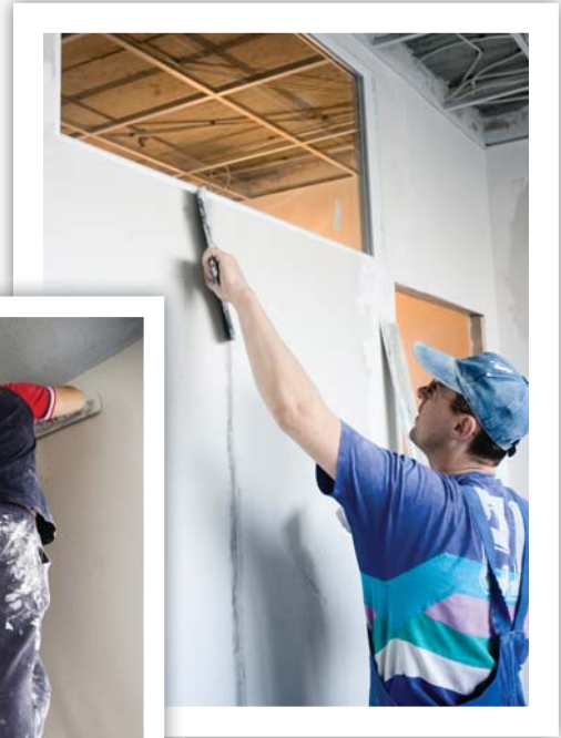
Plastering the board joints in partitions (above) and the junctions of wall and ceiling (left).
