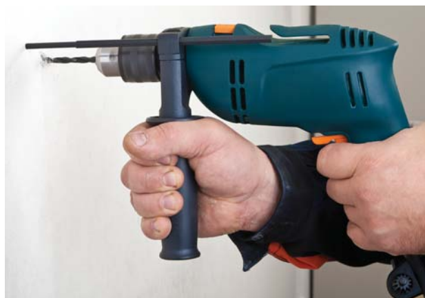
Drilling with power drill
