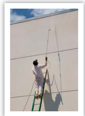
Water or oil based paints applied on pre installed Promat boards.
