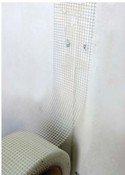
Fill joint with single, thin layer of plaster and then overlay reinforcing mesh.
