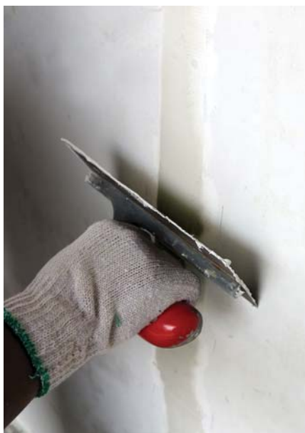
Apply subsequent covering of plaster compound to finish.
