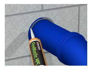
• The sealant can be tooled and smoothed with a pallet knife using water.
